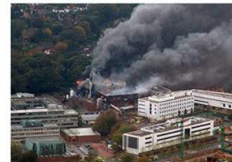
Electronics and Laser Research Building, University of Southampton, 2005
